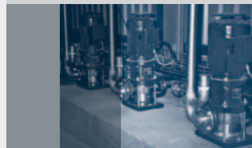
AKV pumps with mechanical seal for pumping chemicals in tank farms.
