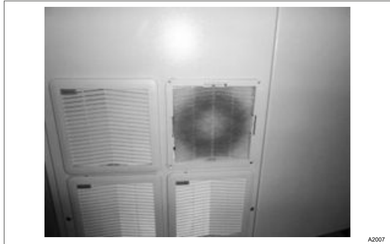
Fig. 39: Cleaning the filters
