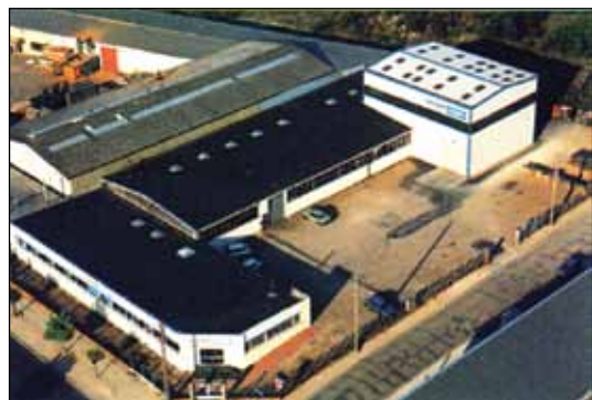
Assembling and Service Center – Orleans, France
