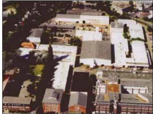
Headquarters and Design Center for Submersible Motors – Hamburg, Germany
