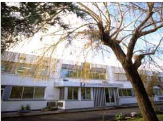
Manufacturing, Assembling and Service Center – Arganda, Spain
