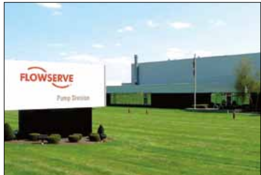
Submersible Motor Center of Excellence (MCO) – Maryland, USA
