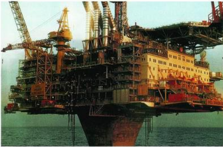
Offshore platform in the North Sea equipped with Pleuger Worthington auxiliary pumps
